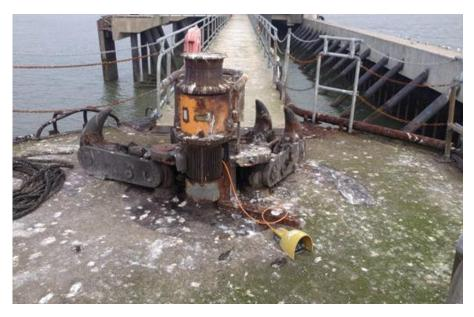
This foot switch for actuating a winch on a mooring hook is continually exposed to saltwater, fouling and seagull droppings – and yet functions perfectly.
